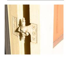
**CLARK'S TIP HINGES** are nearly identical in operation to Acme, Lull & Porter hinges but are surface-mounted.
